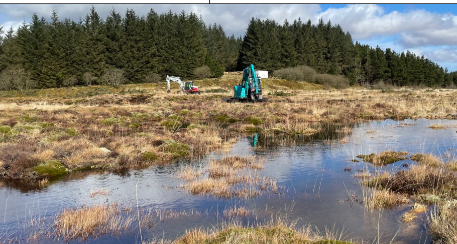
Dealing with eroding peatland at Carn Fflur, in the Tywi Forest region which is part of the Welsh Government Woodland Estate in mid-Wales, the restoration action included re-wetting with low peat dams to create more open habitat for aquatic sphagnum, invertebrates and other species ©National Peatland Action Programme
